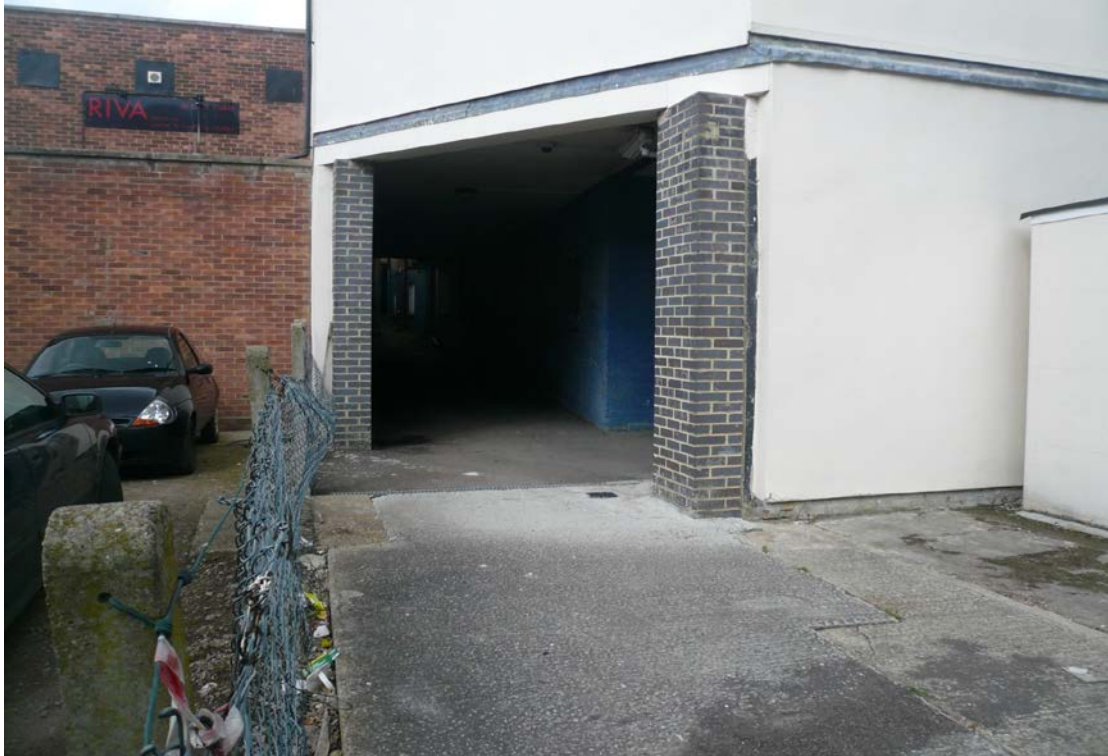
Photograph 3: View of entrance to Shop 25 storage area
